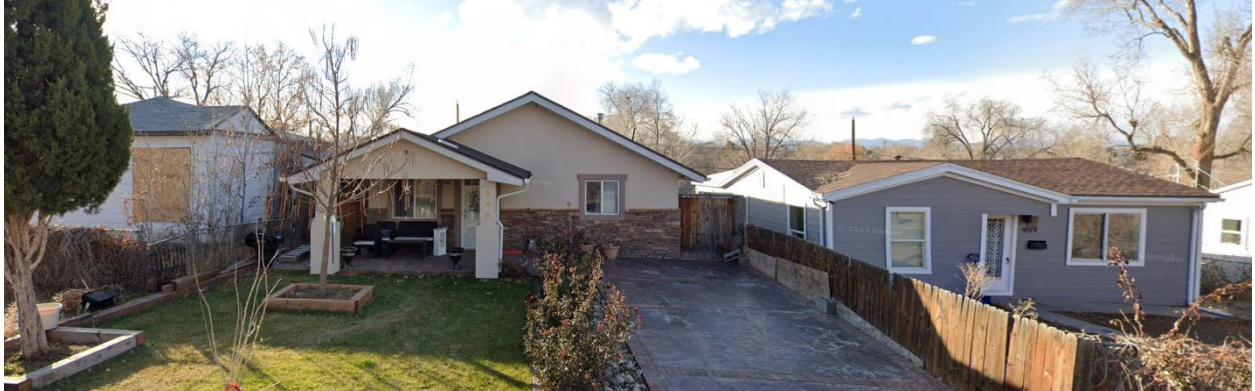
North – View of single-unit properties directly north of the subject site.
