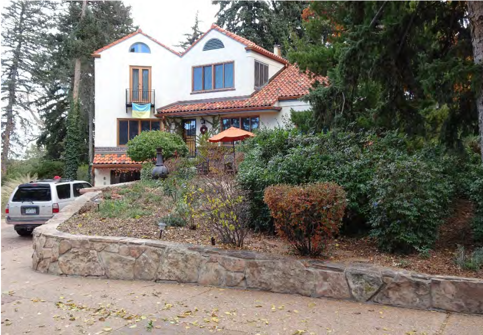
Kunsmiller House west elevation, facing east. Rubble stone retaining wall with concrete cap lines the driveway, and is a contributing historic feature. Square Moon photograph 2022.
