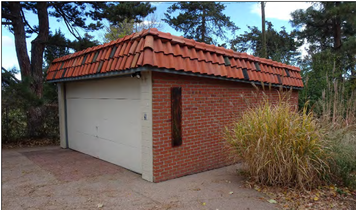
Kunsmiller House Garage, c. 1978, facing northwest. This is a noncontributing feature to the historic property. Square Moon photograph 2022.
