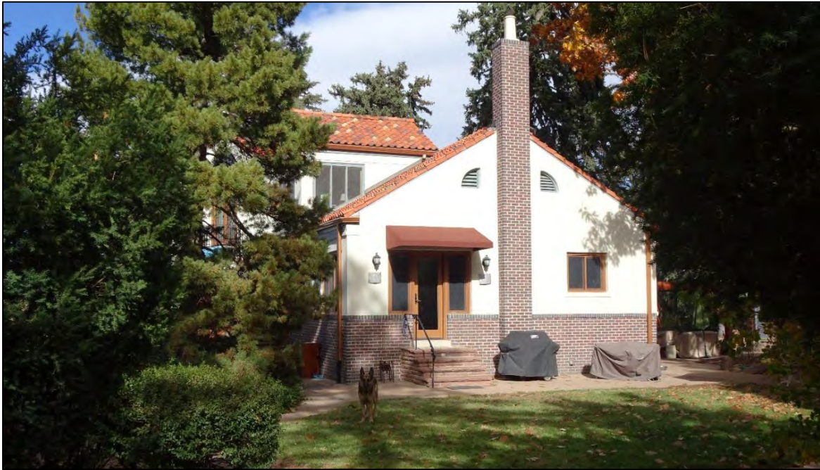
Kunsmiller House south elevation, facing north-northeast. Square Moon photograph 2022.
