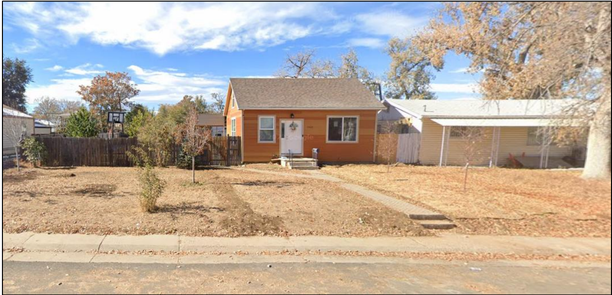
View of the subject property looking west from N. Verbena St.
