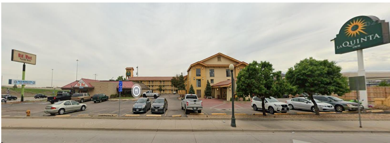
View of the subject properties, looking east.
