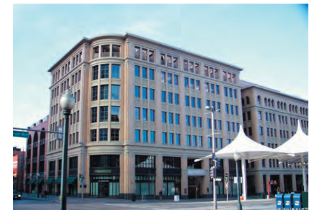
New building in LoDo reflects general desired characteristics of the anticipated guidelines.
