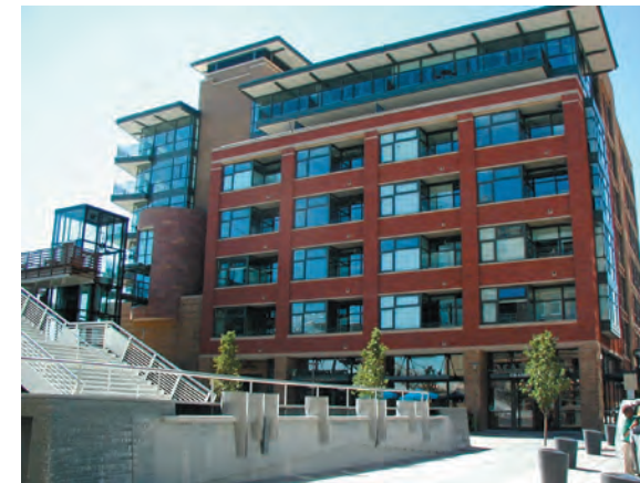
Promenade Lofts at Riverfront Plaza, with ground-level retail/office.
