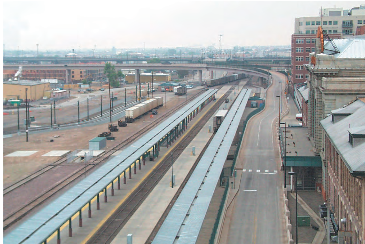
View of Station Platforms looking northeast. Note 20 th Street HOV ramp and flyover, ca. 2003.
