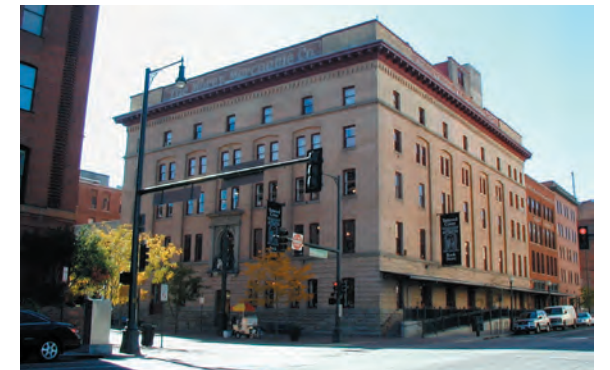
Adaptive reuse in LoDo with first three floors retail (Tattered Cover Bookstore) and residential lofts above.
