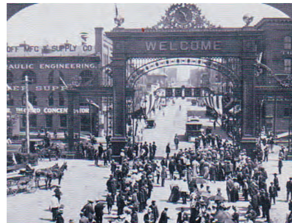
Welcome Arch, looking southeast up 17 th Street.
