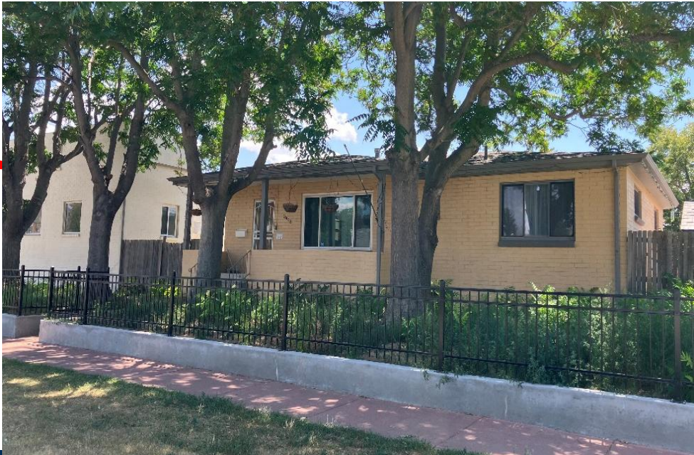
Subject property: 3418 W. 14th Ave (view from 14th Ave facing southeast)
