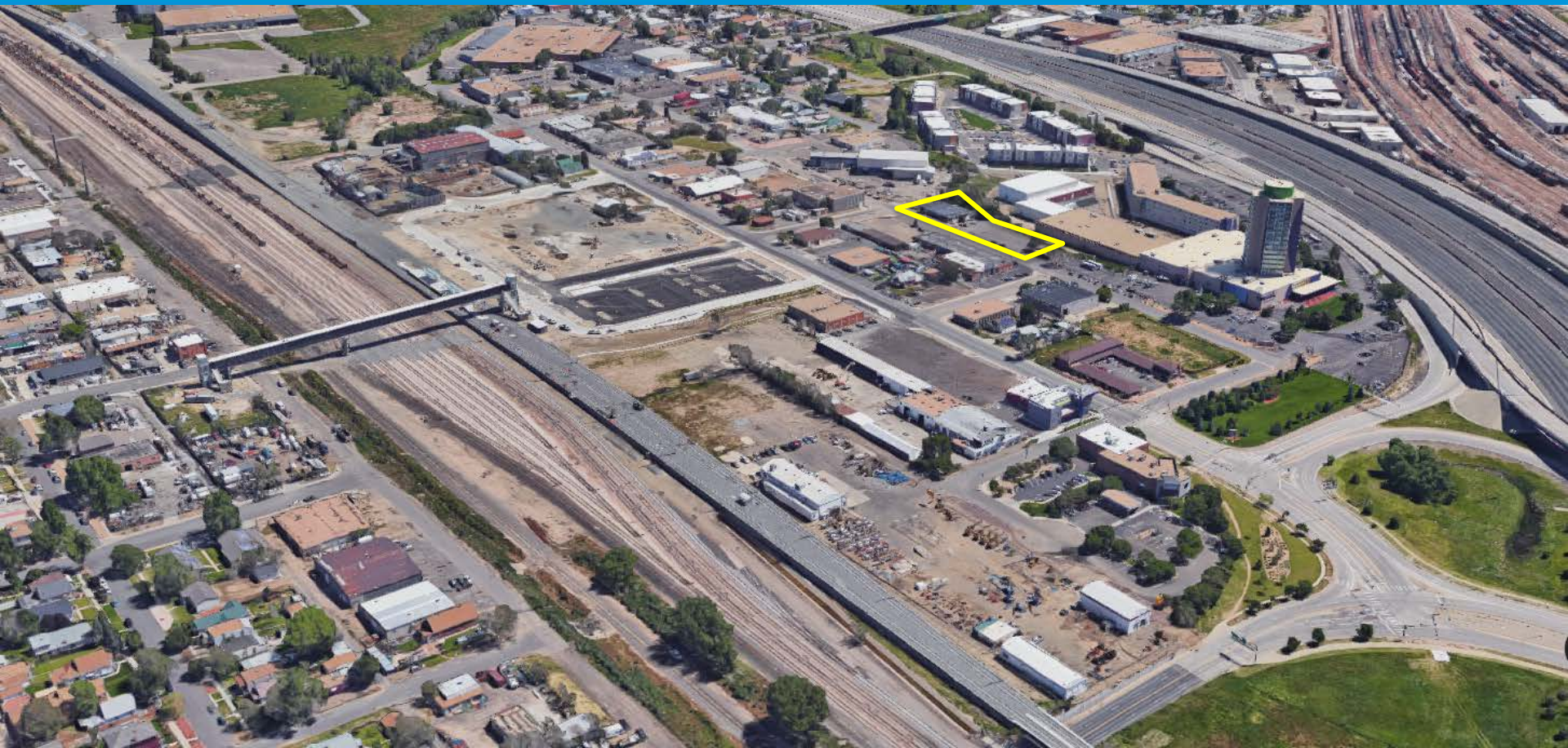
Aerial, looking northeast (Google Maps)
