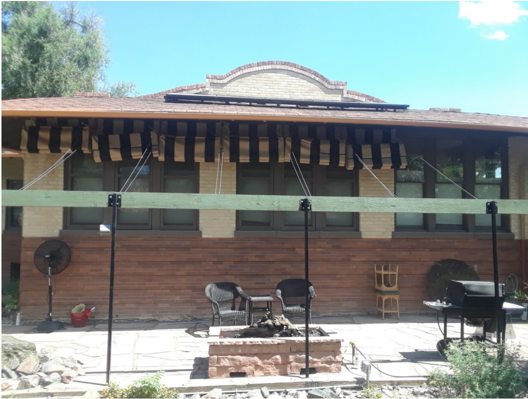
Figure 2 Enclosed "cure porch" on the west elevation
