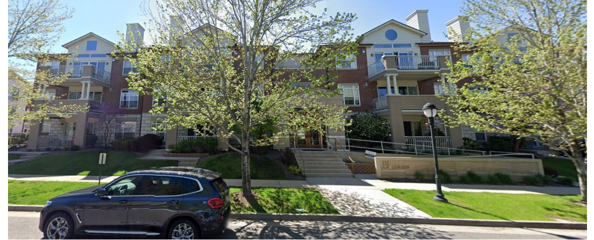
Looking east on Monroe Street south of Bayaud Avenue
