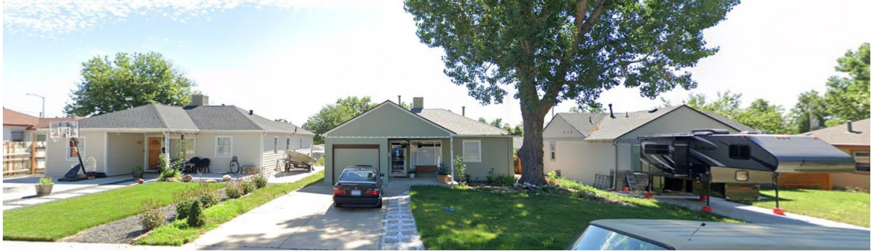
View of the 4740, 4750 and 4758 Clay properties, looking east.
