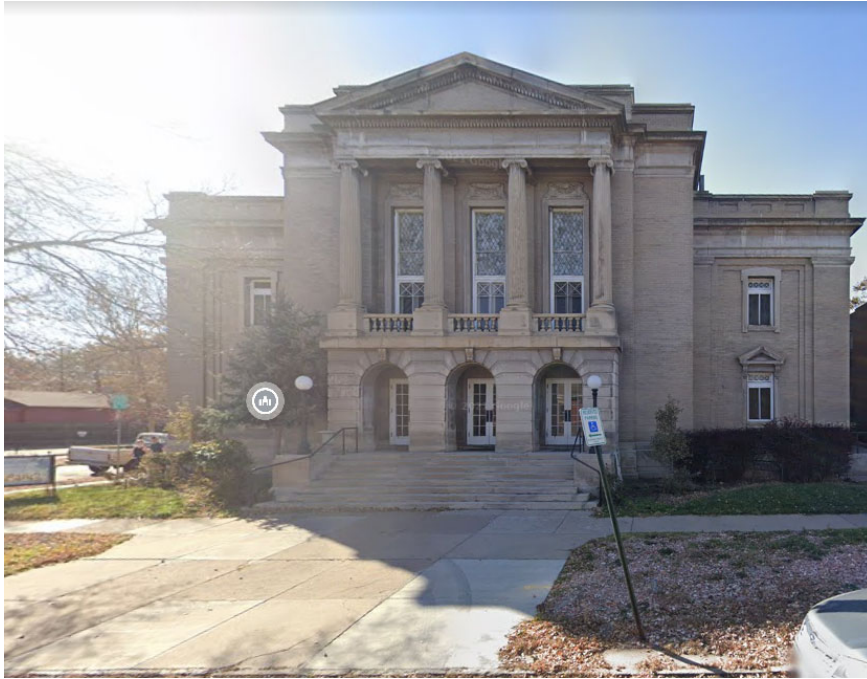
Site: Looking west from South Grant Street.
