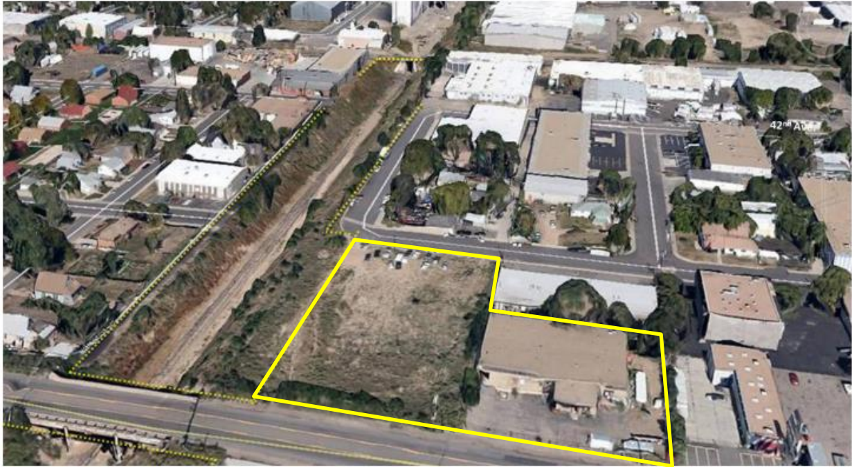
Market Lead underpass existing condition
