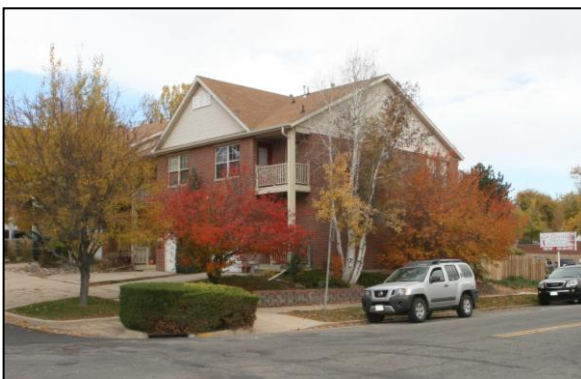
New Apartment 29 th Avenue and Yates Street
