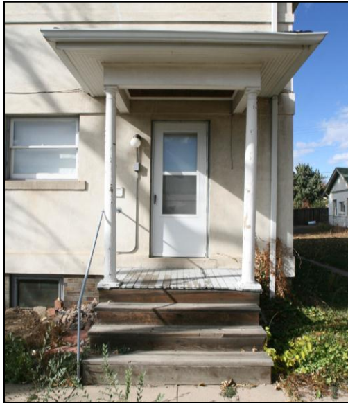
East Elevation, North End, Replacement Porch, Looking West
