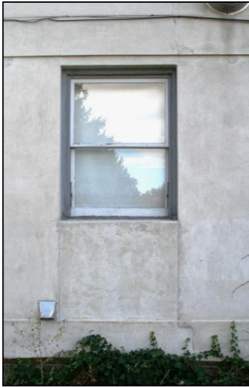
North Elevation, Door turned into a window
