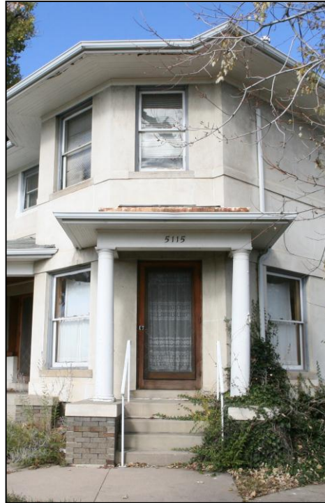
Southeast Corner, Looking Northwest
