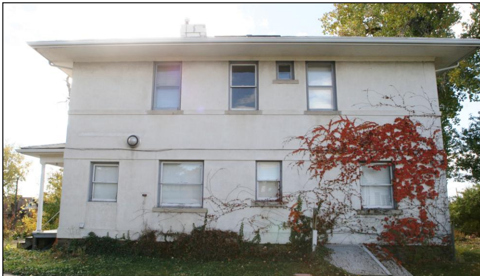
North Elevation, Looking South
