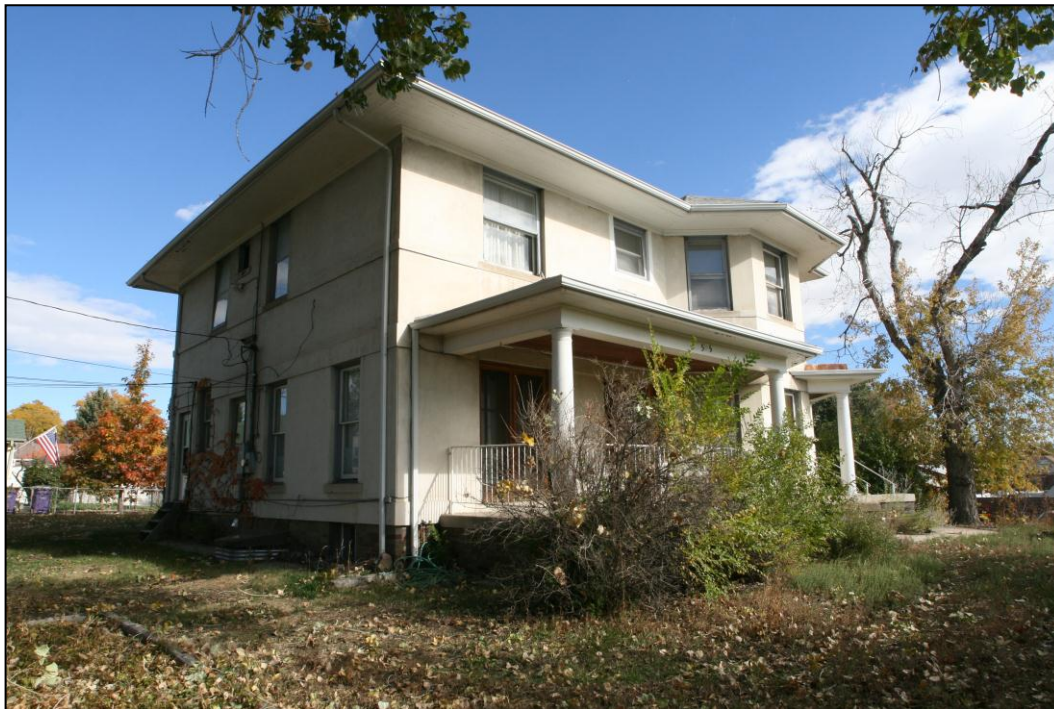
South Elevation, Looking Northeast from the Southwest Corner of the Lot
