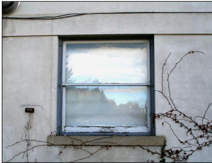
North Elevation, Replacement Window – Typical of the House
