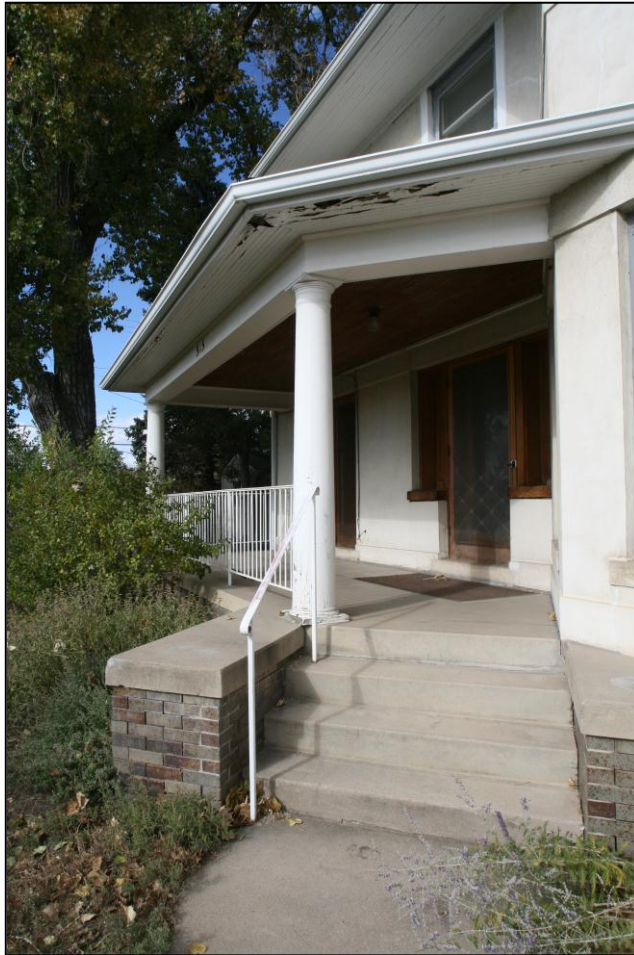
South Elevation, Porch, Looking Northwest from the Walkway
