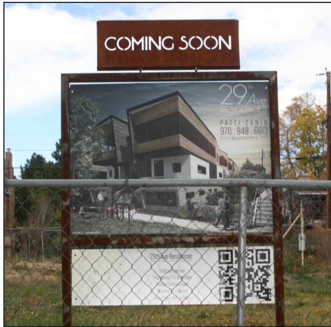
Proposed New Apartments on vacant land at 29 th Avenue and Yates Street
