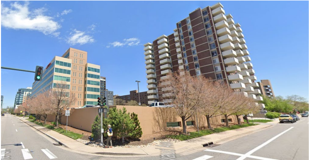
View facing northeast from the corner of Steele Street and Bayaud Avenue
