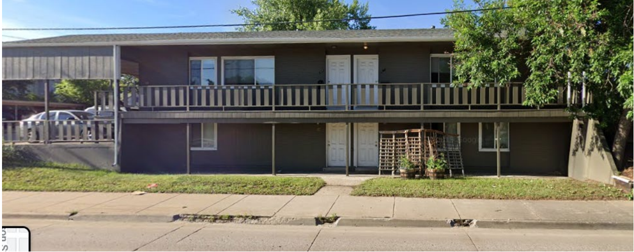
View of the property to the north looking south.
