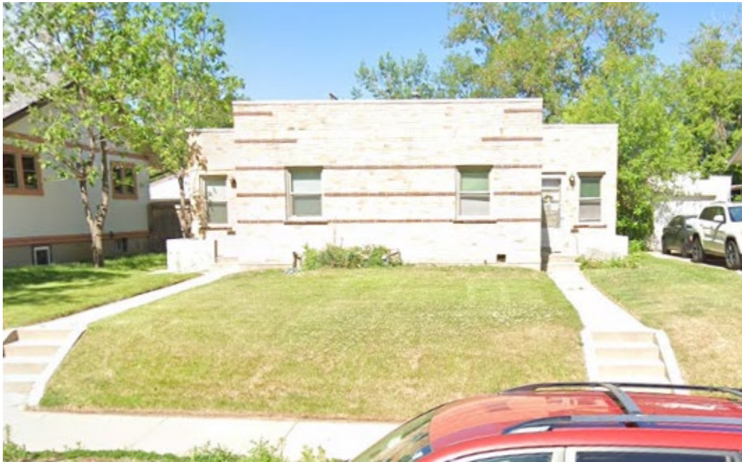
View of the property to the west across S. Emerson St., looking west.
