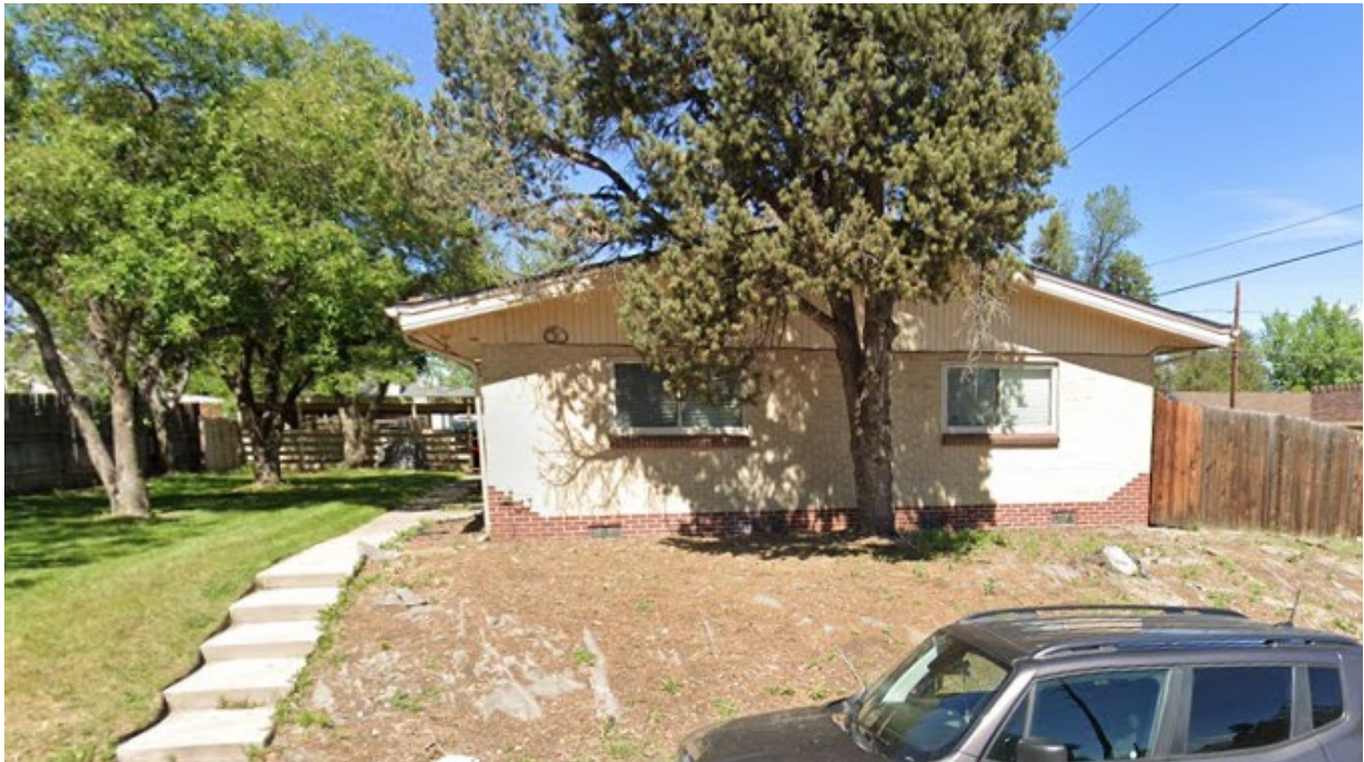
View of the property to the east across the alley, looking west.
