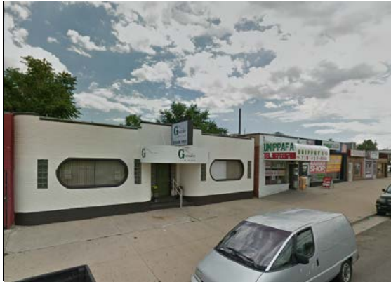
Commercial structures north of subject property
