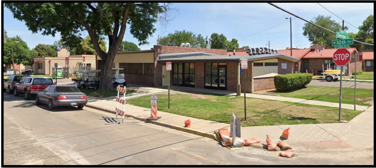
Buildings typical of DHA Sun Valley Homes – from Decatur St and 10 th Avenue (Source: Google Maps)
