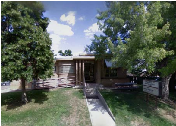
Legal non-conforming clinic north of the subject property
