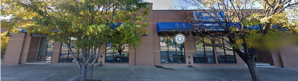
View facing south on Colfax Avenue between Glencoe Street and Grape Street – near the proposed rezoning area
