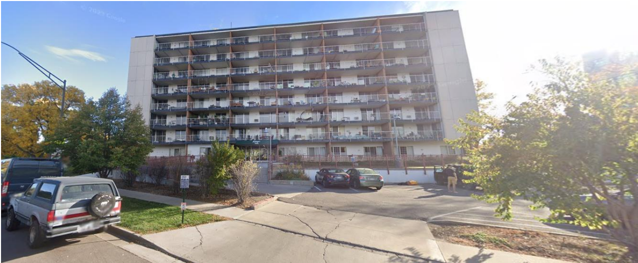
View facing south on Hale Parkway between Dahlia Street and Eudora Street – near the proposed rezoning area
