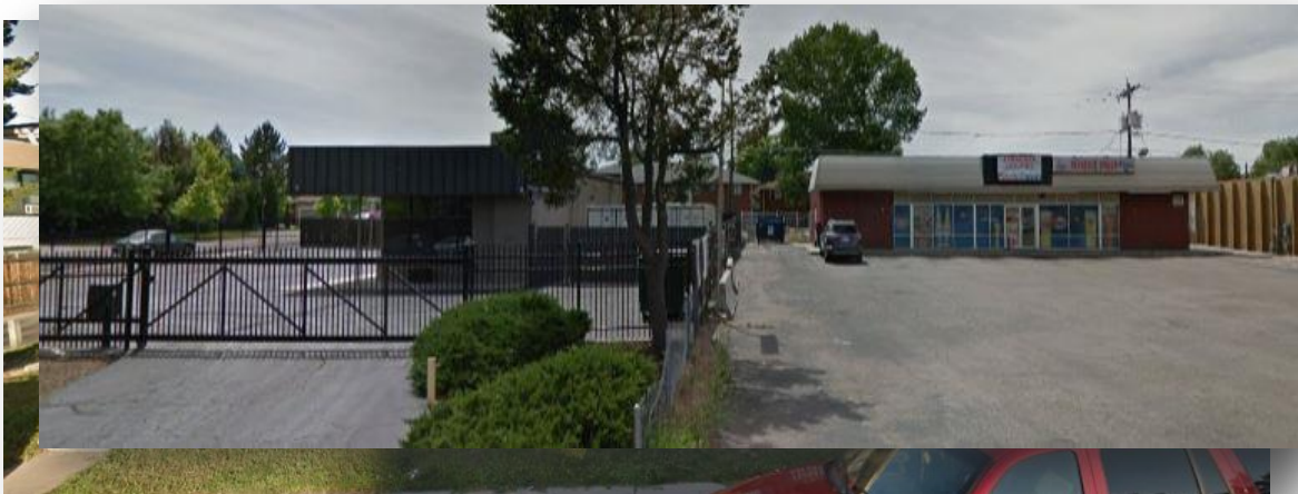
Figure 6: 1100 Block Syracuse St. (Commercial Property Center)
