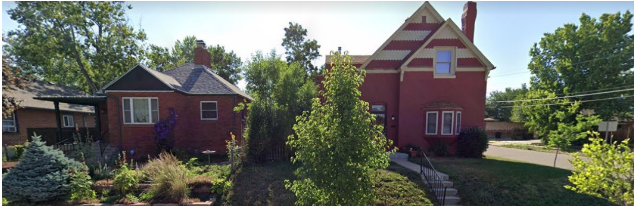
View facing west on King Street north of 27 th Avenue – within proposed rezoning (U-SU-B)
