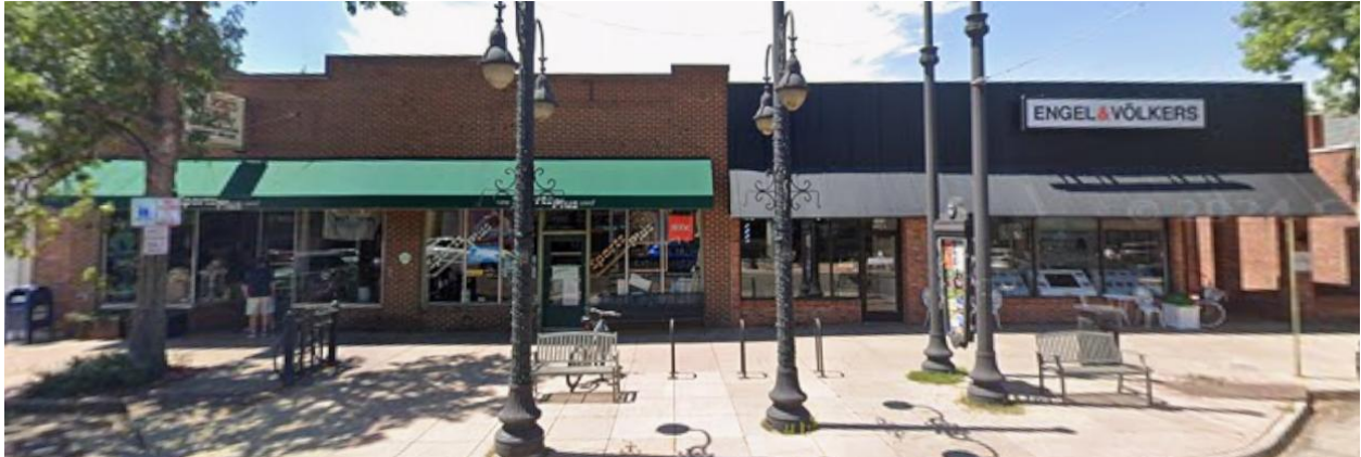
View of properties to the north of the subject property along S Gaylord Street looking west.
