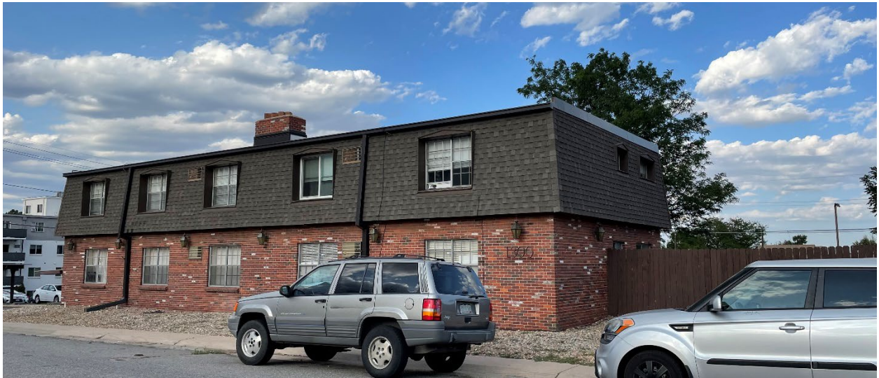
North end of block face: Looking northeast from South Birch Street.
