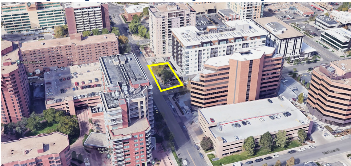
Aerial view, subject property highlighted, looking northwest
