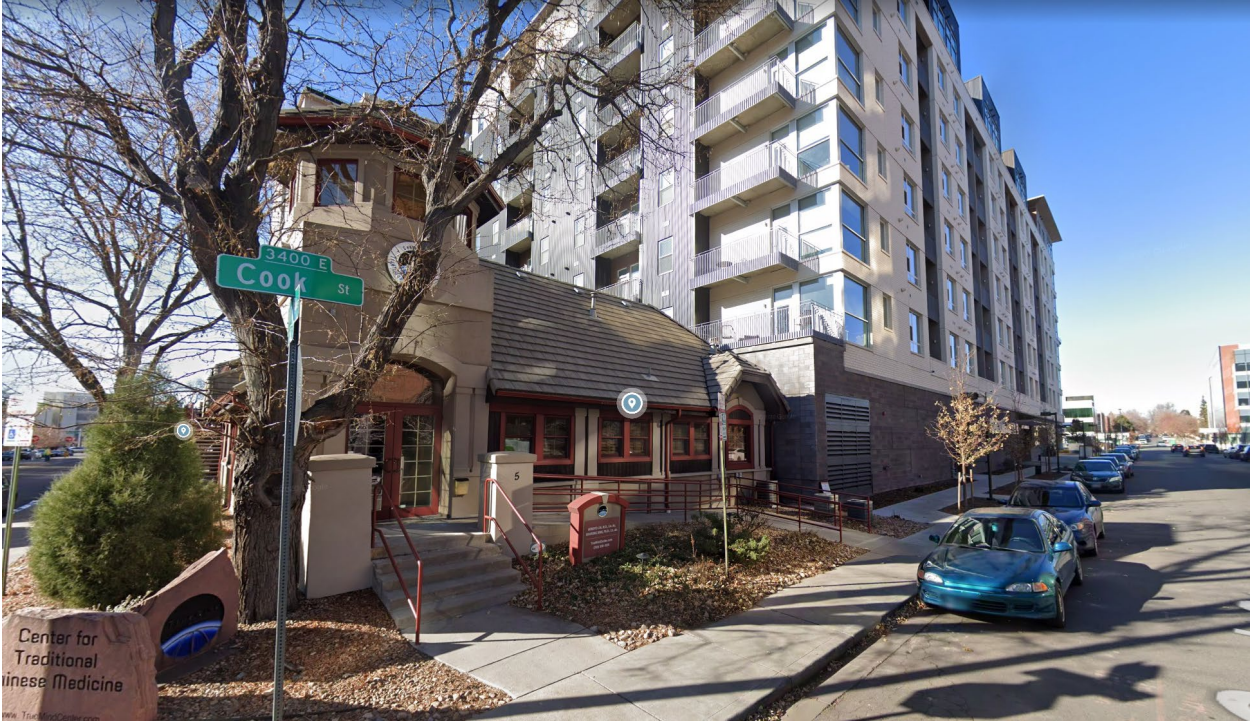
Subject site facing east on Cook Street
