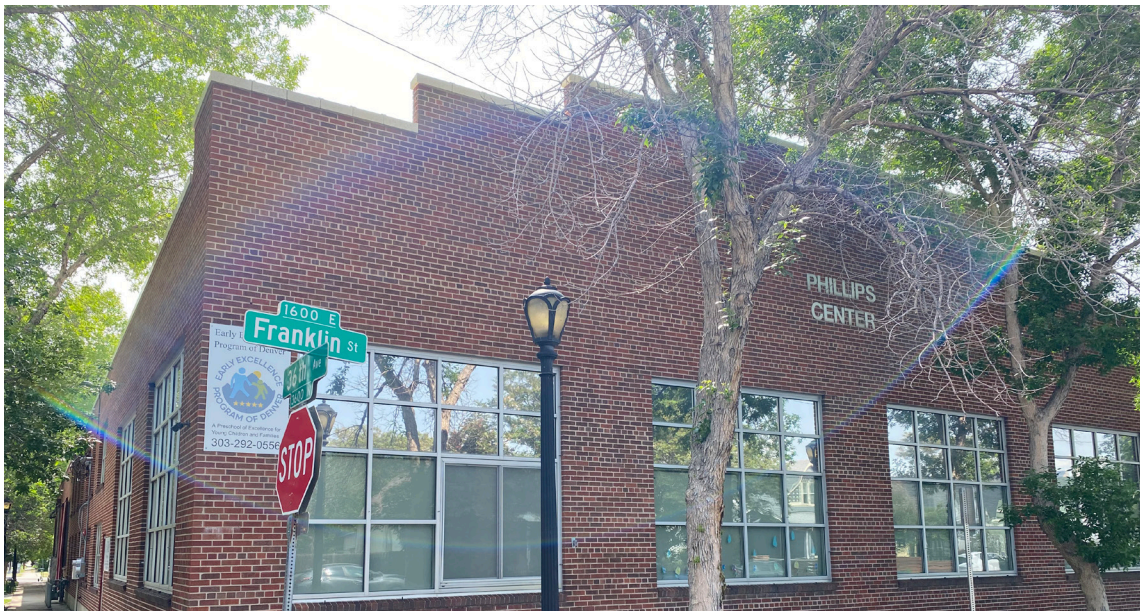
Figure 1-3 Existing West elevation, with red brick, parapet and stone cap, and divided light windows. Not to Scale. Illustrative Only.
