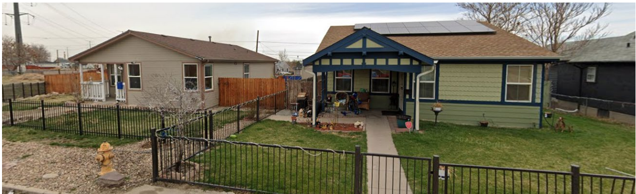
View of properties to the north of 4748 N Leaf Ct, looking east from Leaf Ct
