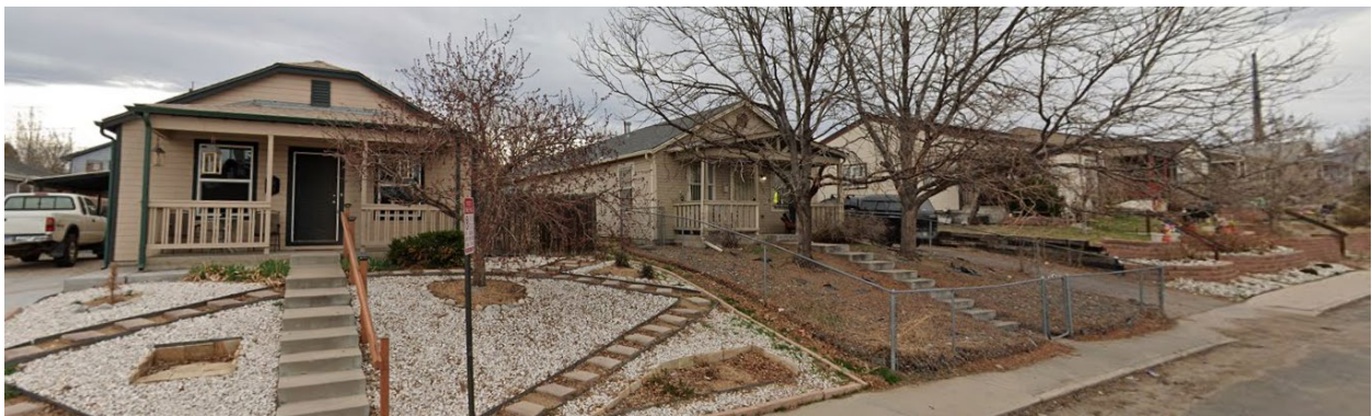
View of the property to the west of 4710 N Lincoln St, looking west from Lincoln St
