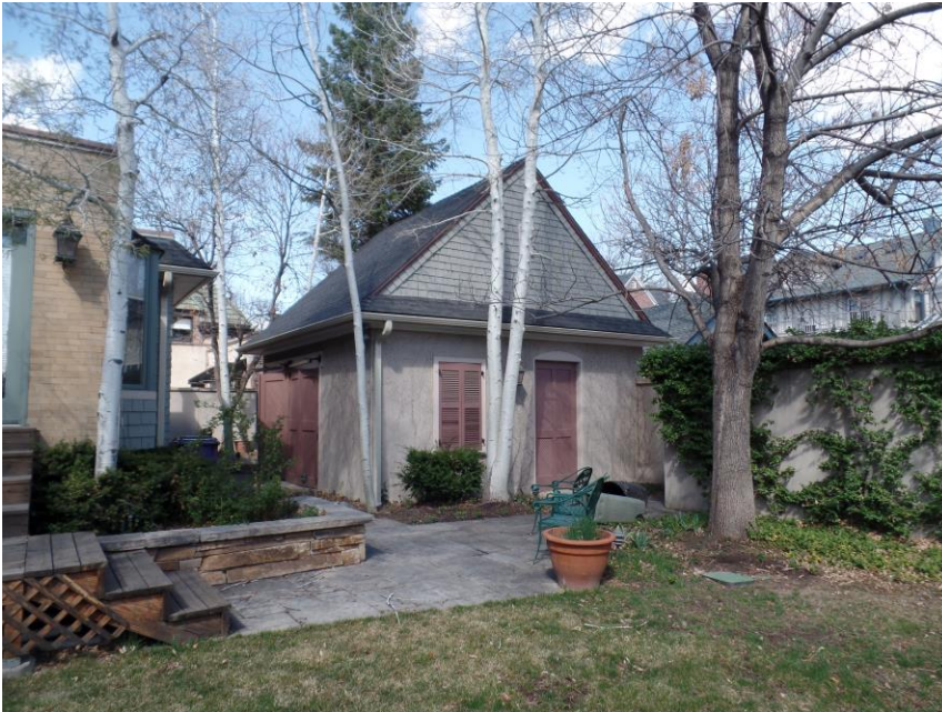
Carriage house from the south
