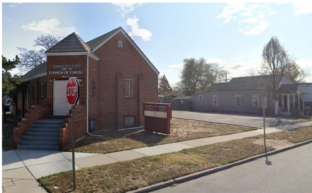
West – from Clayton St. & 44 th Ave. Source: Google Maps
