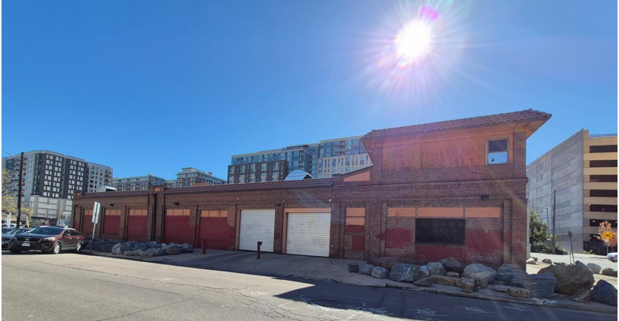
California Street Garage, northwest elevation (2025)
