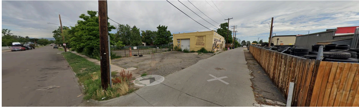
View of property to the east, looking northwest.
