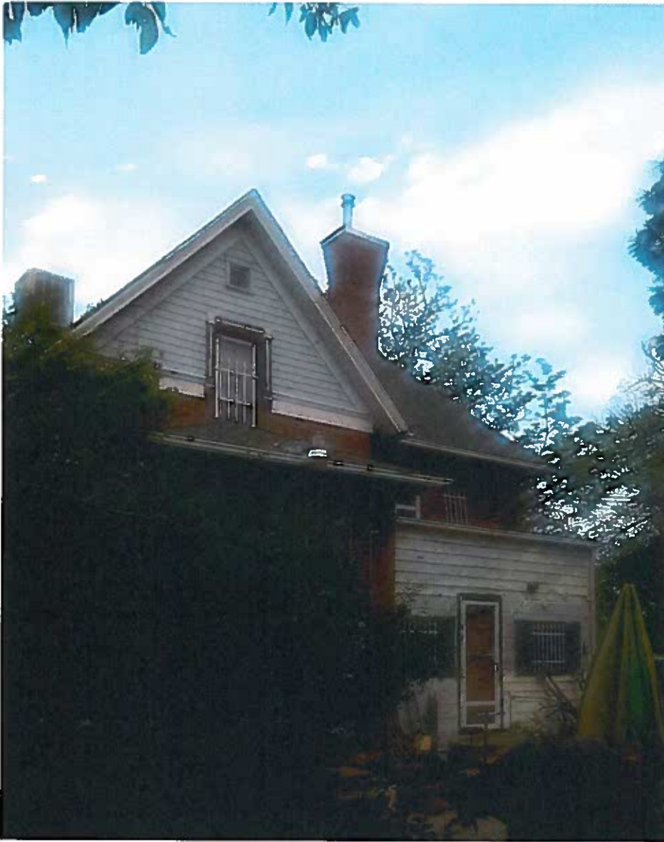
The western elevation of the property, which faces into the carriage lot. Note the later addition to the back of the building.
