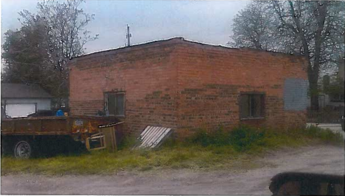
One of the out buildings on the property.
