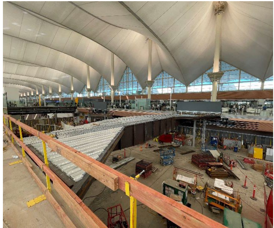
Bridge connecting the East and West Checkpoints is currently being constructed
