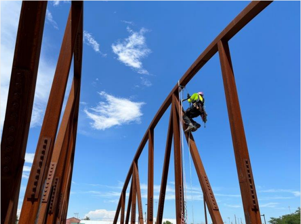
2024 Bridge Inspection Program
