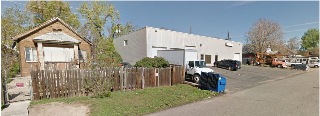
One-story, single family residential structure and one-story industrial building to the south of the subject site, looking north
