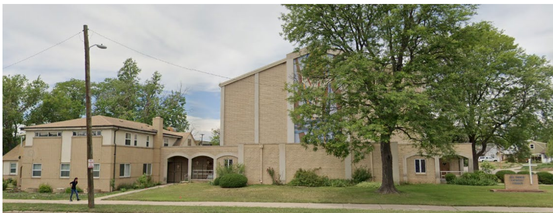
All Saints Church north of the subject site, facing west from S. Federal Boulevard.
