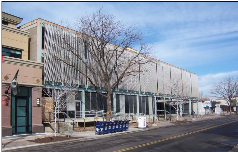
245 Columbine Street, showing existing 3-story structure to the south and 1-story structures to the north.
