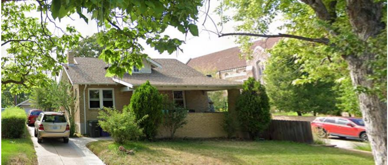
North – from Eudora Street looking west
