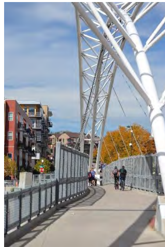
Left: Looking north across the Highlands Pedestrian Bridge.
