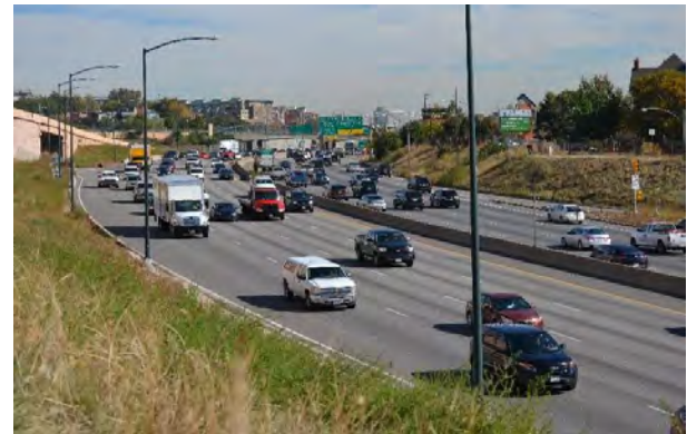
I-25 looking north from the 23rd Avenue bridge
