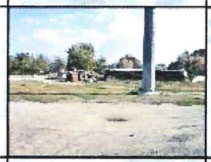
2 EXISTING CONDITIONS: VIEWS FROM THE NORTH
