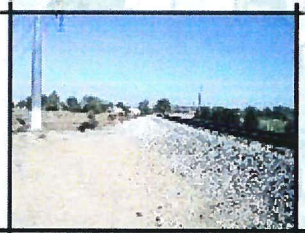
4 EXISTING CONDITIONS: VIEWS ALONG THE RAIL ROAD TRACKS
