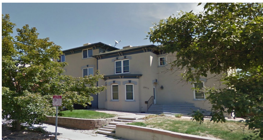
Two-story house directly west of the subject site, facing east from N. Vallejo Street.
