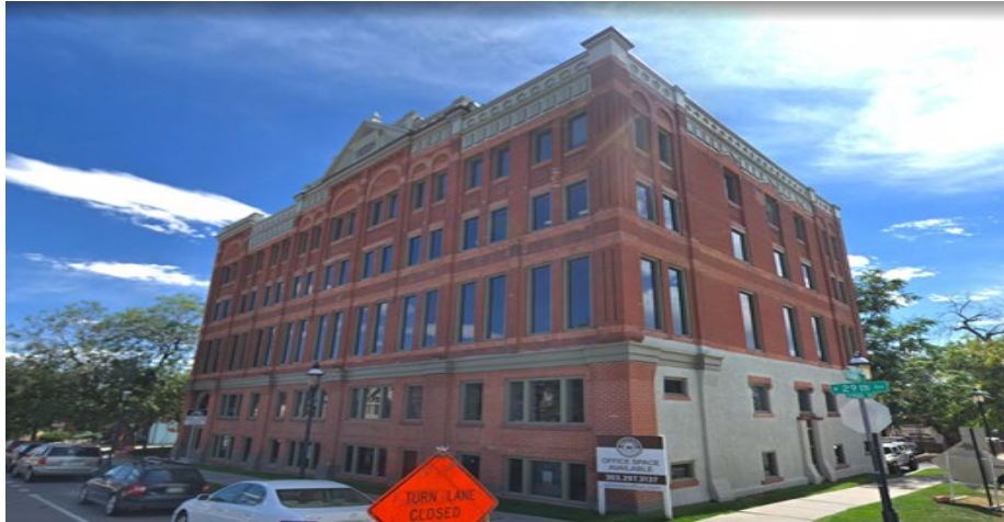
Five-story office building directly south of the subject site, facing southeast from W. 29 th Avenue
