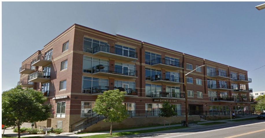
Four-story mixed-use development southwest of the subject site, facing southwest on W. 29 th Avenue.
