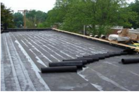
Built-up Roof (BUR)
