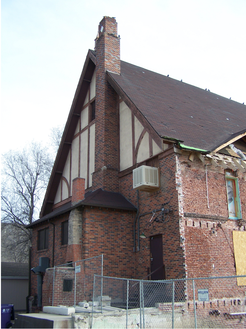
Photograph 5. The West façade of the 1931 structure.
