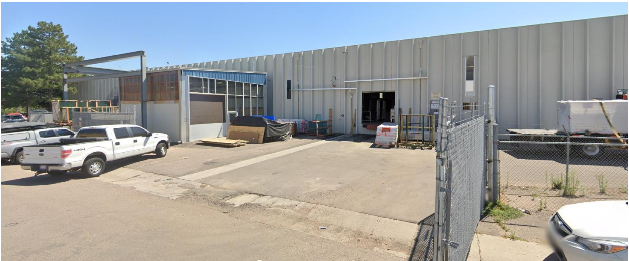
East – from South Fox Street (Source: Google Maps)
