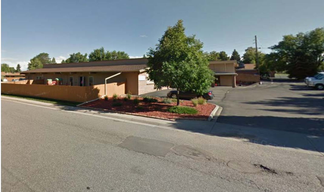
Subject property; view from West Vassar Ave (source: Google maps)
