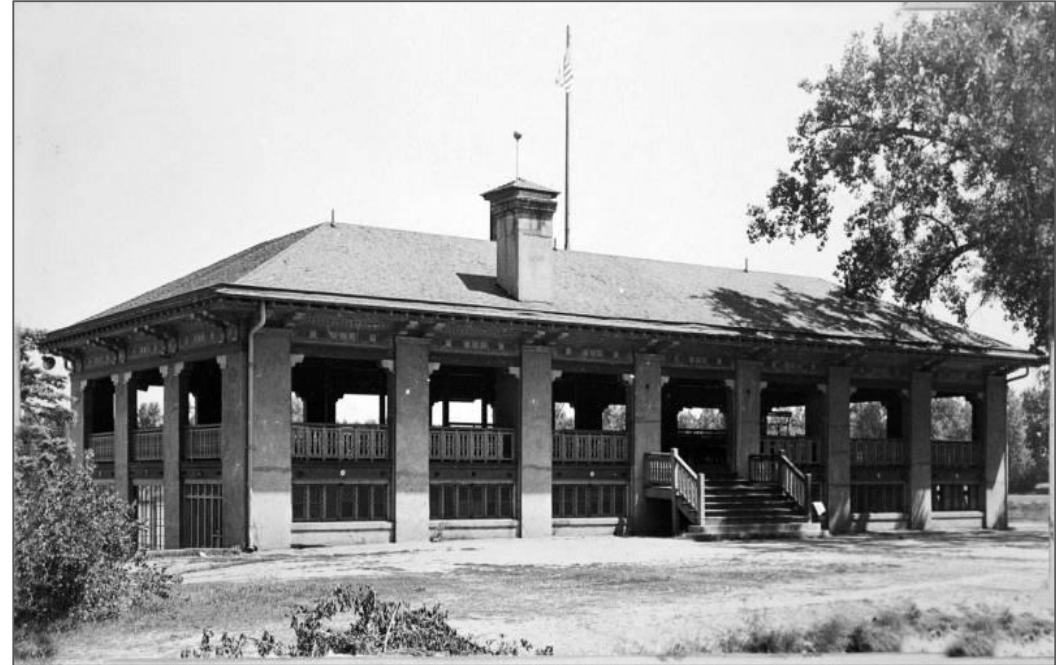
Benedict-designed boathouse in Washington Park (Source: Denver Public Library Digital Collections)
