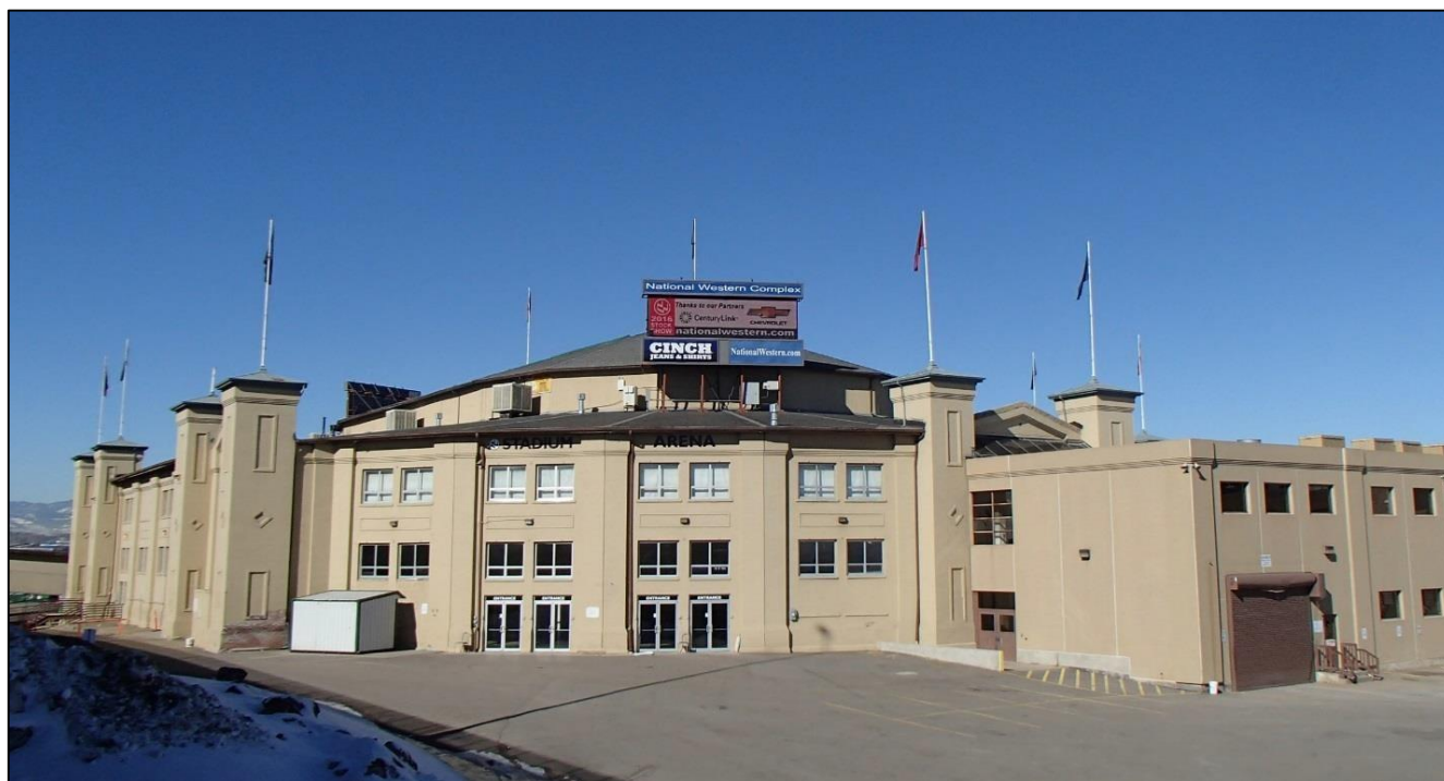
Stadium Arena, East Elevation Photographed by Kathleen Corbett February 9, 2016
