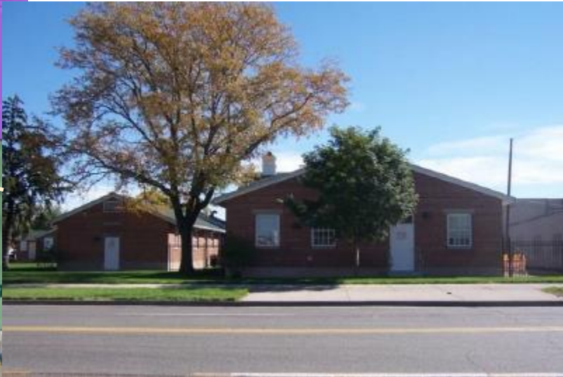
Inner City Health Center looking east
