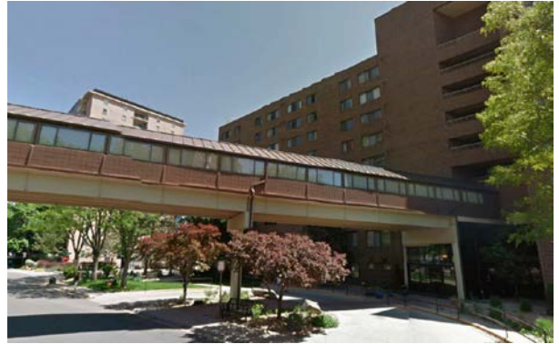
Subject site looking north and east down South Adams Street towards the second-story enclosed pedestrian bridge that connects 44 South Adams Street to 11 South Adams Street (not visible)
