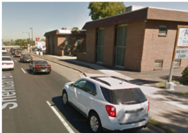
Subject site; looking north
