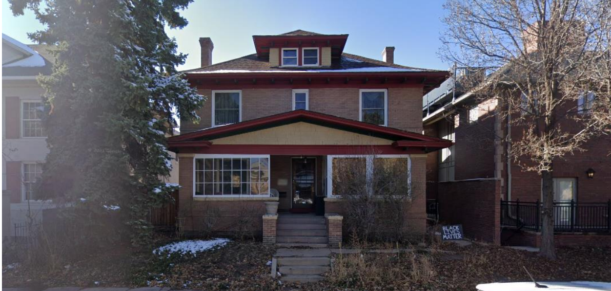
South – the property to the south, from North Clarkson Street facing west (Source: Google Maps)
